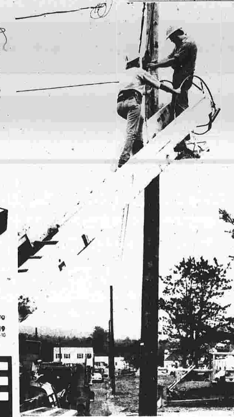
Two Southern New England telephone company workers cut in phones for new houses on Wellman Road. Left: Sandy Lance of 24A Sycamore Lane and Al Krob of 119 Porter St.
